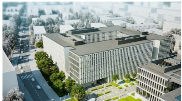
Name of building: Office building Bobrowiecka 8 Country: Poland City: Warsaw Units: VENTUS
