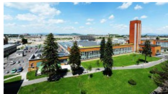
Name of building: Coresi Business Park Country: Romania City: Brasov Devices: VENTUS
