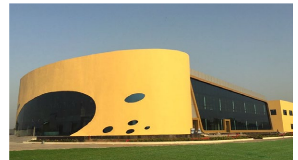
Name of building: JDM House Country: India City: Vadodara Devices: VENTUS
