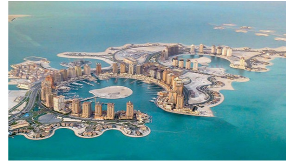
Name of building: Moon Island-Pearl Qatar Country: Qatar City: Doha Devices: American VENTUS
