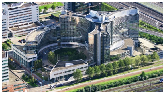
Name of building: Park Inn Hotel Country: Netherlands City: Amsterdam Devices: VENTUS
