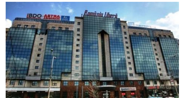
Name of building: City Business Center Country: Rumunia City: Bucharest Devices: VENTUS
