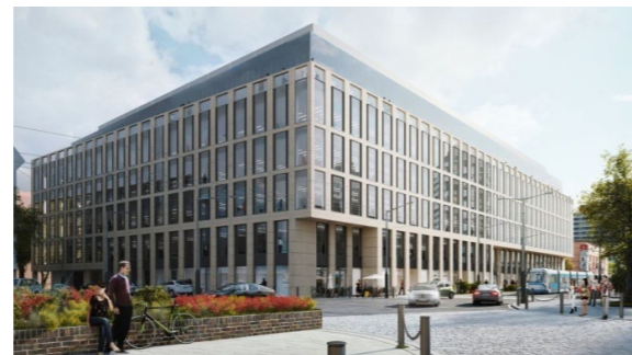
Name of building: Nobilis Business House Country: Poland City: Wroclaw Devices: VENTUS
