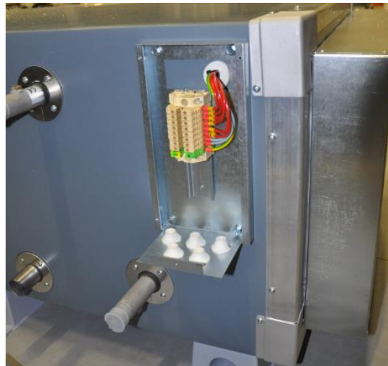
Fig. 17 Layout of electric heater's terminal block.
