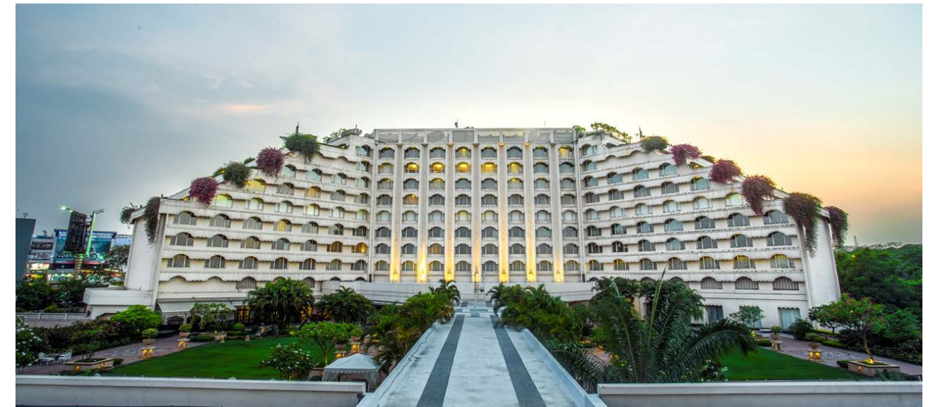
Name of building: Taj Krishna Hotel Country: Indie City: Hyderabad
