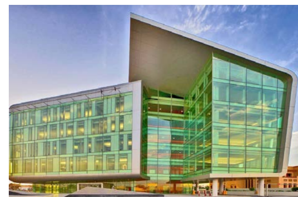
Name of building: Emiarates Telecommunication Corp Country: UAE Abu Dhabi City: Abu Dhabi
