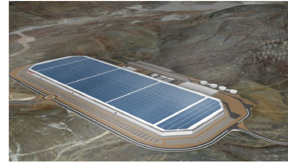
Building name: TESLA Gigafactory Country: USA City: Sparks Devices: American VENTUS
