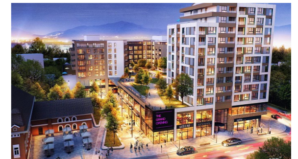
Building name: Platinia Malle Country: Romania City: Cluj Napoca Devices: VENTUS
