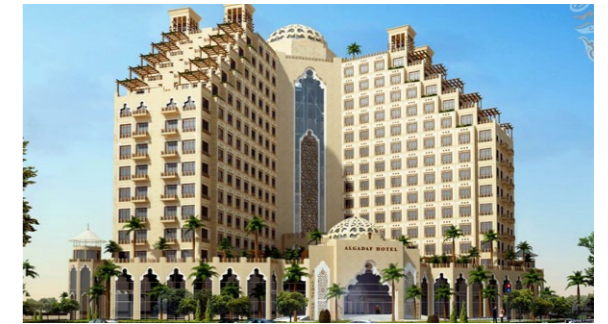
Building name: Residential and Commercial building B+G+1P+12T in Al Jadaf Country: Dubai City: UAE Devices: VENTUS
