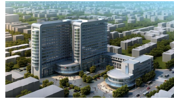
Building name: The traditional Chinese Medicine Hospital Country: China City: Inner Mongolia, Hohhot Devices: VENTUS
