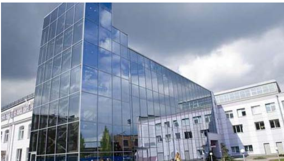
Name of building: Kondratievsky Business Center Country: Russia City: Saint Petersburg Devices: VENTUS
