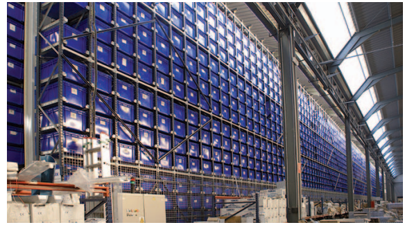
Name of building: SECOM SA Country: Romania City: Chiajna Devices: WING
