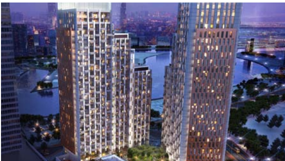
Name of building: The Atria Tower Country: UAE City: Dubaj Devices: VENTUS
