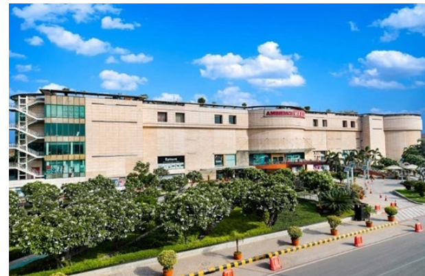
Name of the building: Ambience Mall at Vasant Kunj Country: India City: Delhi
