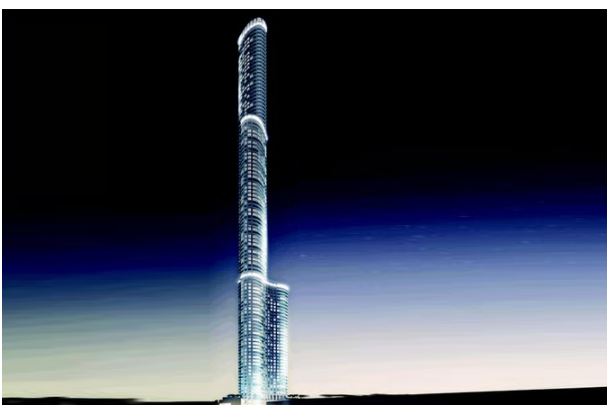
Name of the building: Lodha World One - Prince Tower Country: India City: Mumbai
