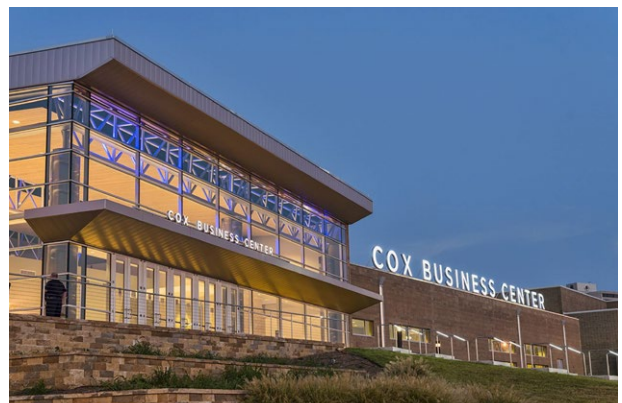
Name of the building: Cox Business Center Country: USA City: Tulsa, OK
