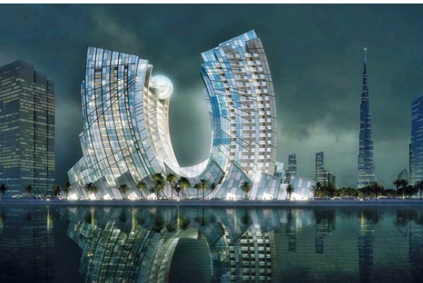
Name of the building: Residential Complex (J One Tower) Country: UAE City: Dubai
