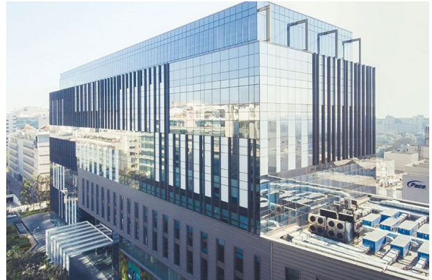
Name of the building: Samsung Manyata Tech Park Country: India City: Bangalore
