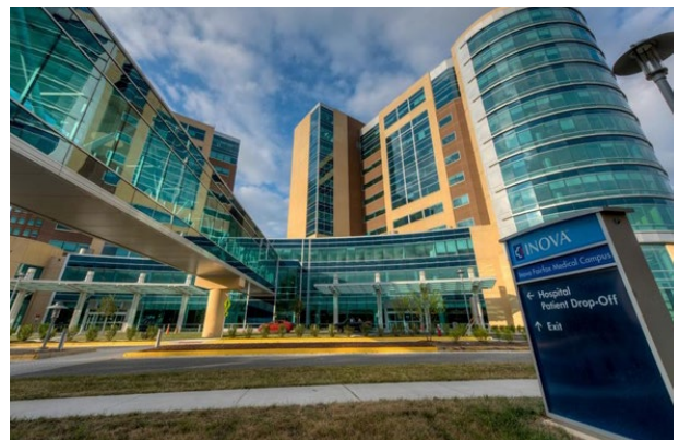
Name of the building: Inova - ATS Country: USA City: Falls Church
