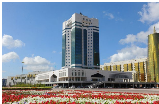
Name of the building: The Government House of the Republic of Kazakhstan Country: Kazakhstan City: Nur-Sultan
