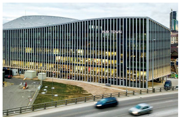
Name of the building: Office Center Park Town Country: Lithuania City: Vilnius
