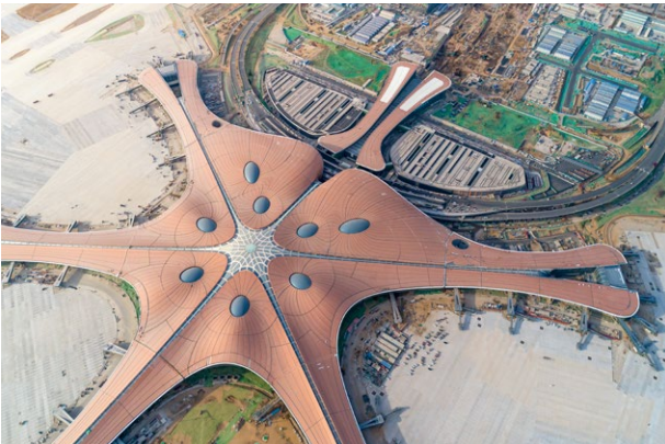
Name of the building: Daxing Airport Country: China City: Beijing
